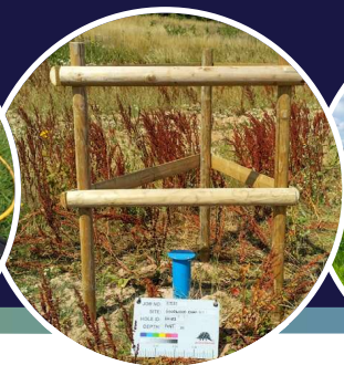
Groundwater and gas monitoring
